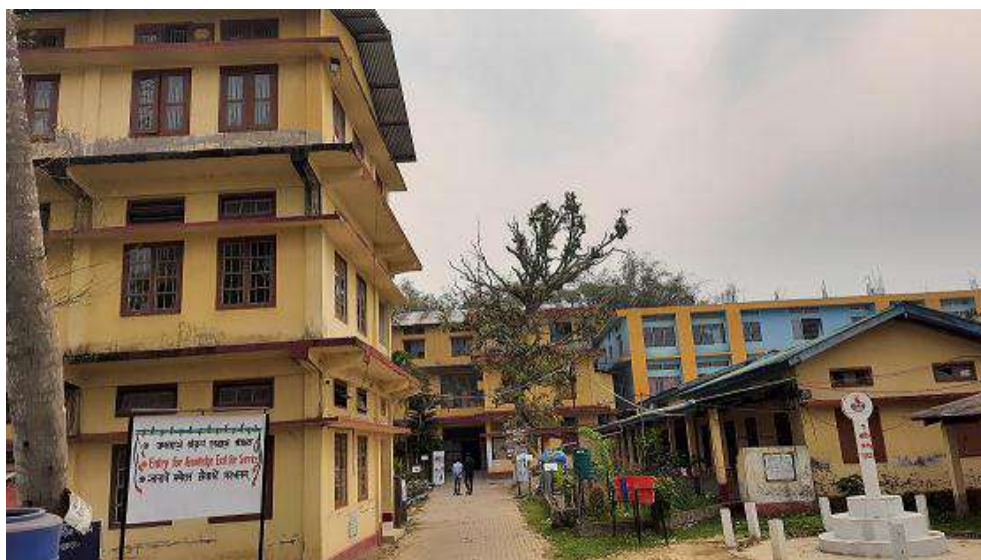
Photo 1: Snap shot of the building
